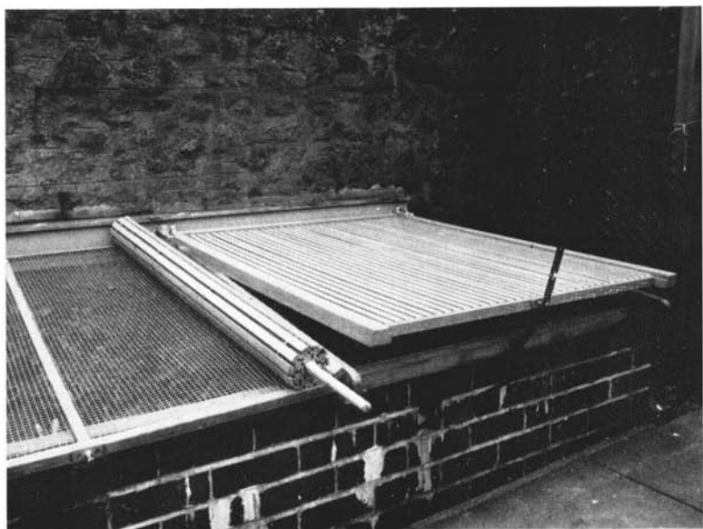
Fig. 13—Pit Frames with Wire Mesh Grilles (see page 82)
